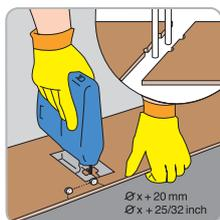
If you have heating pipes, measure their exact position and mark it on the laminate. Add 20mm to the dimension of the pipe, because the laminate has to be able to move in all directions around the pipe. Saw from the drilling holes to the side of the laminate in an angle of 45° and put the laminate in place.
